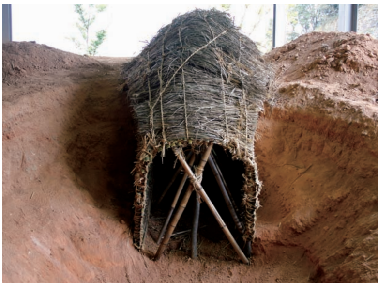
Method 1: Set up wood pillars at the center of the floor and make an arched ceiling by bending bamboos.
