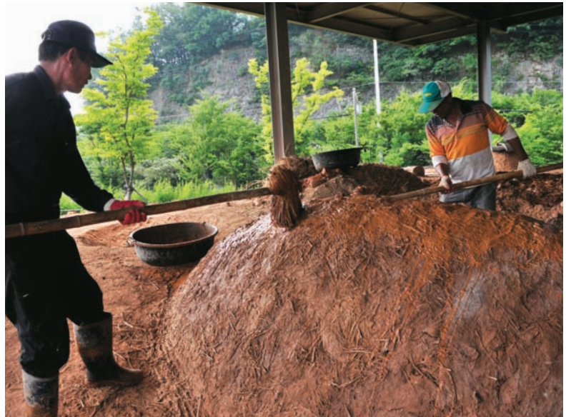
Cover the kiln ceiling frame evenly with mud.
