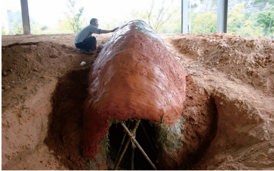
Applying clay on the ceiling frame meticulously several times
