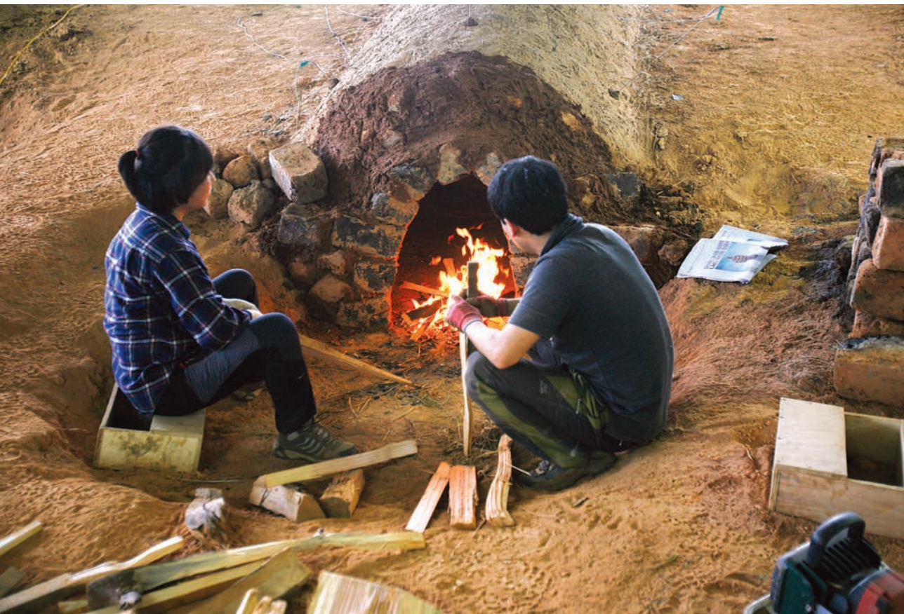
Assistant Researcher Lee, Hye-won and Assistant Researcher Gang, Myeong-seok making a starting fire to dehumidify the inside of the kiln
