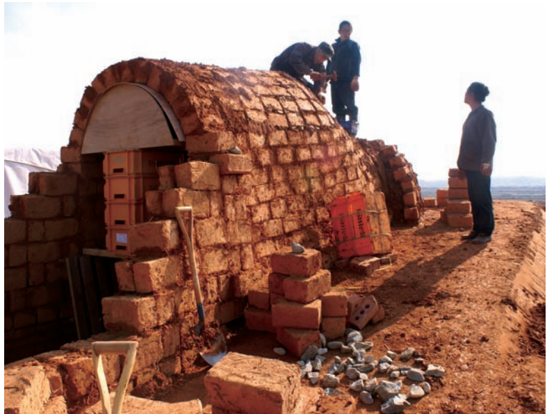
The first kiln was made with soil bricks, led by Master Onggi Artisan Lee, Hyun-bae.
