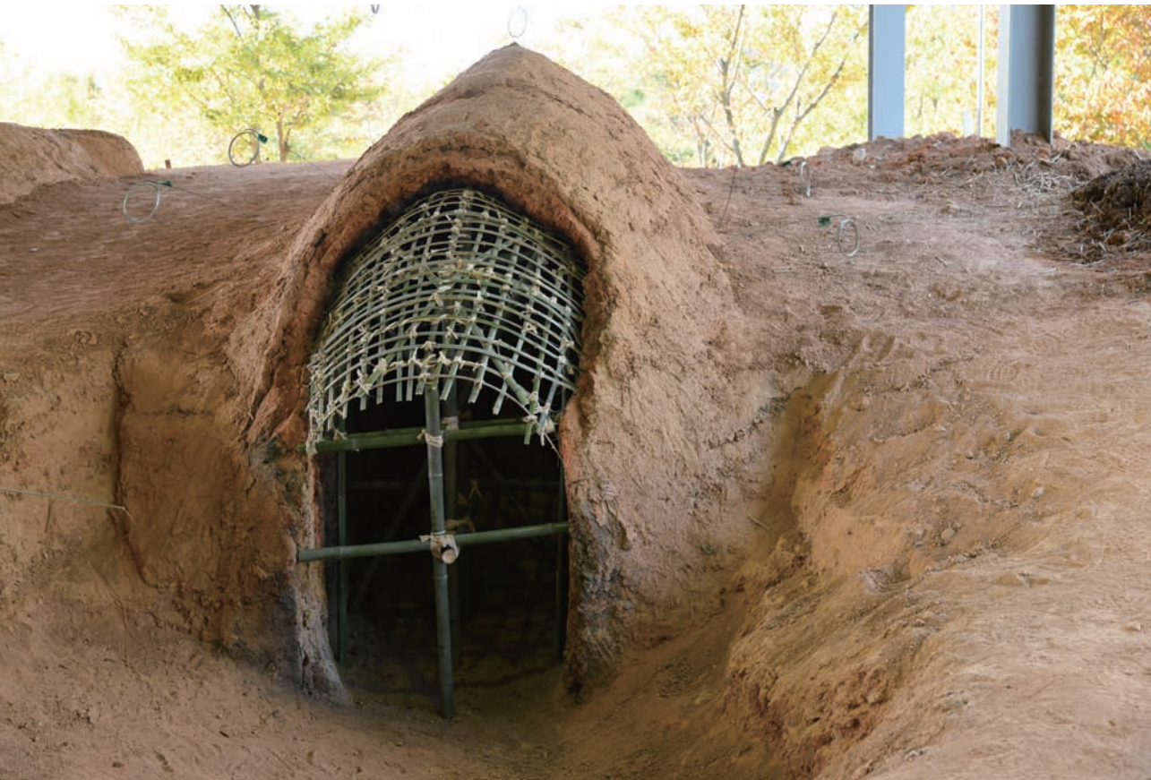
Bamboo frame on the combustion chamber ceiling
