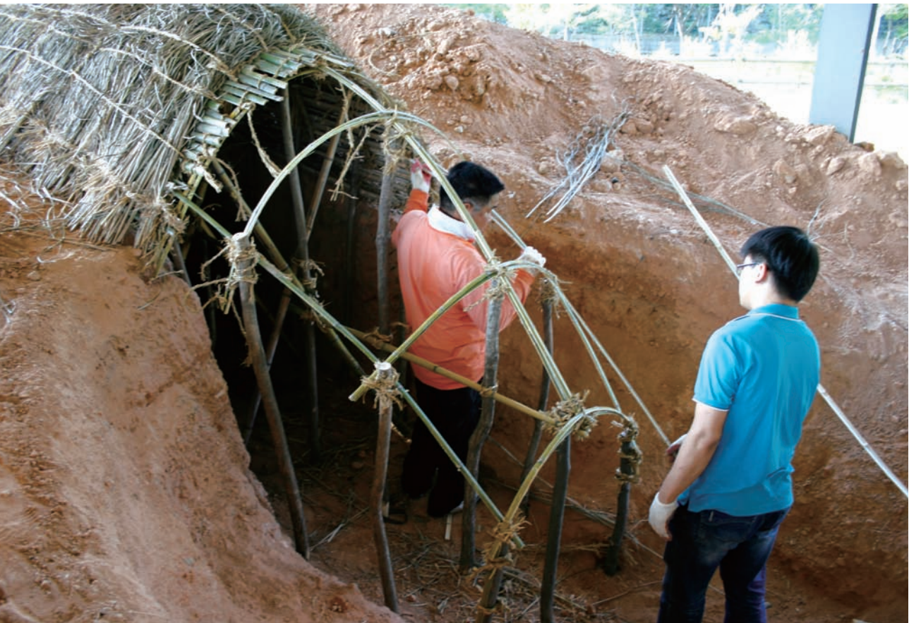
Making an arched ceiling structure using bamboos, led by Researcher Jeon, Yong-ho
