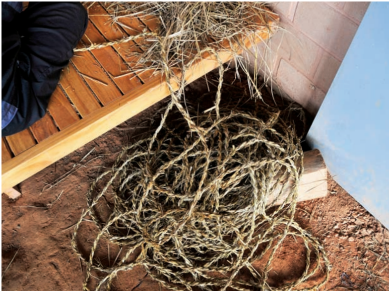
Making straw ropes to connect the kiln frame
