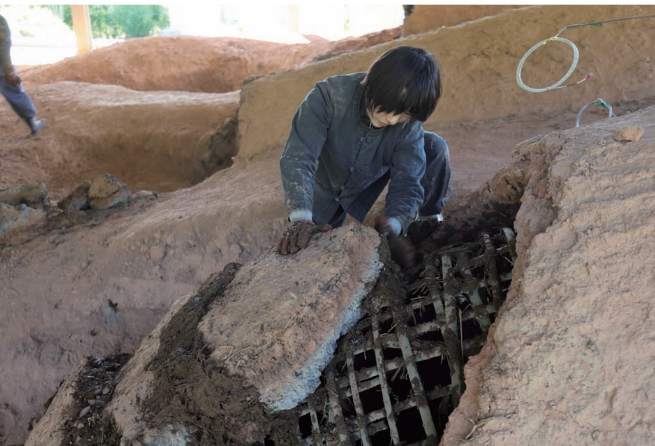
Covering the combustion chamber ceiling using kiln ceiling pieces and mud
